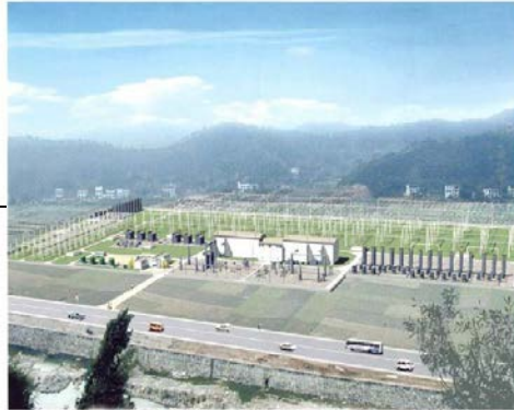
HVDC Converter Station > 6400 MW, Classic
