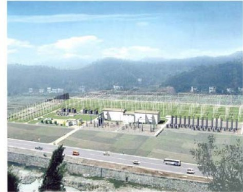
HVDC Converter Station > 6400 MW, Classic
