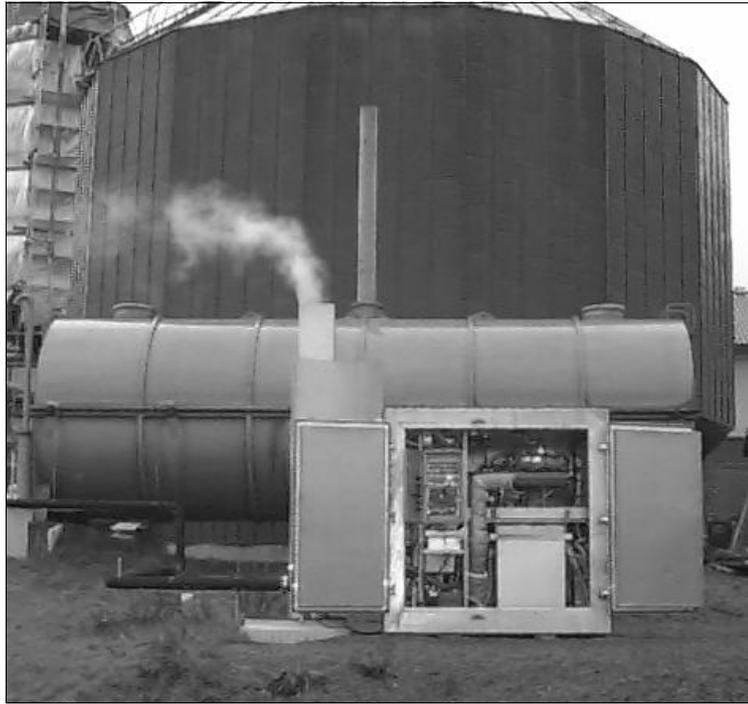
**Figure 2.1** A CHP plant with open doors. The V8 engine is placed in the upper right corner and below it are the heat exchangers. To the left is the control unit cabinet with the door opened, the dark area is the control unit. The work and result of this thesis is the design of this control unit, from design ideas all the way to implementation of a printed circuit board, including functional tests. A more detailed picture of the final result is seen in Figure 5.2.
