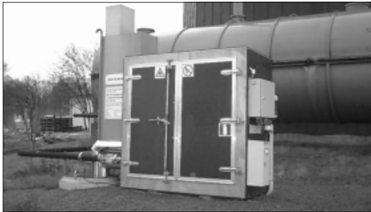
**Figure 2.2** A CHP plant running on digester gas.
